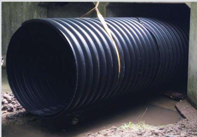
Iowa 72" pipe slip, two runs, 83' lengths
