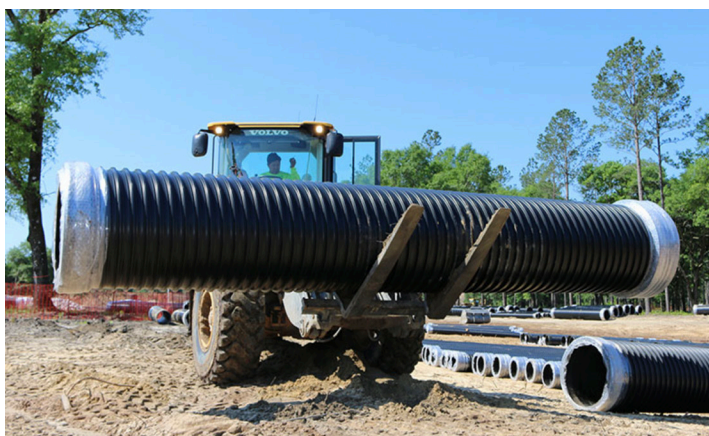
Figure 8 Using a Front-end Loader to Carry Pipe
