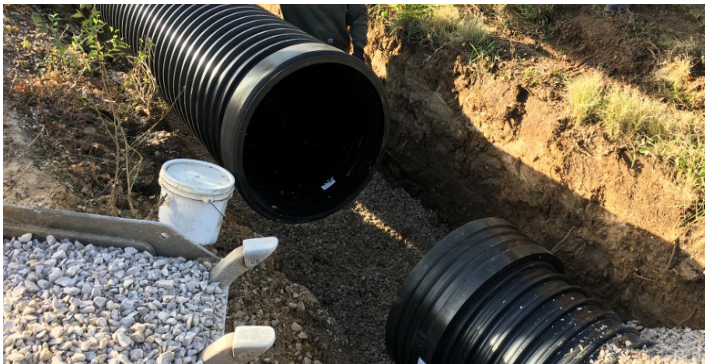
Figure 19 Pipe & Spigot Joint Assembly with Bell Holes
