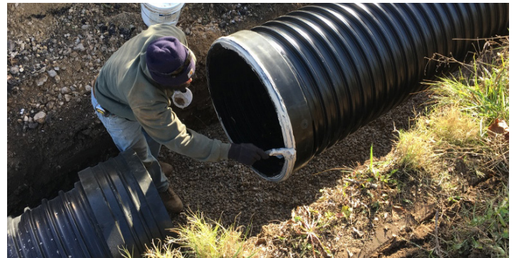
Figure 18 Applying Lubricant to the Joint Spigot Prior to Insertion
