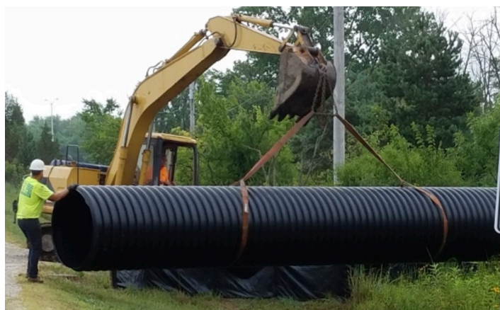
Figure 7 Field Example of Pipe Lifting
